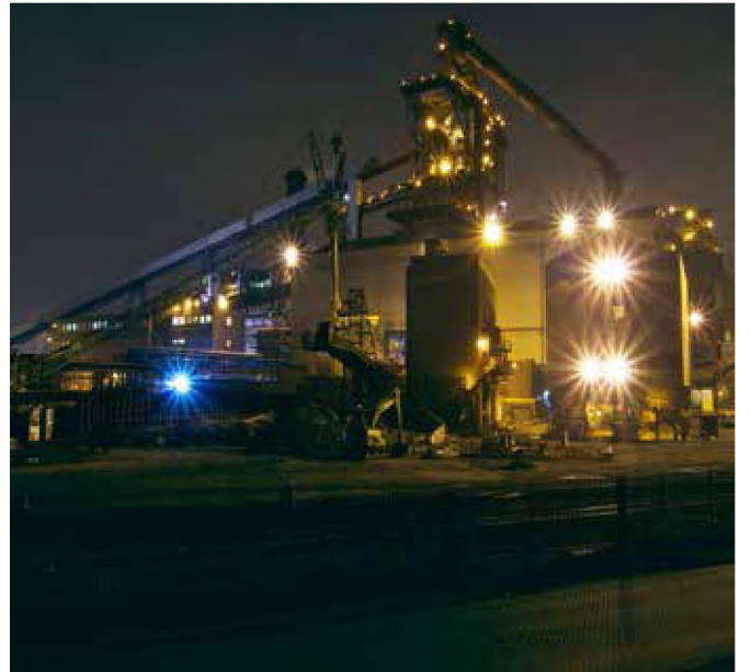
Impianti Industriali / Industrial Equipment / Industrieanlagen
